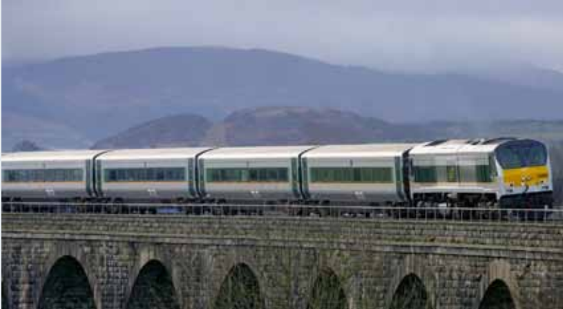
The Dublin-Belfast 'Enterprise' crosses Craigmore Viaduct outside Newry, the highest viaduct in Ireland.
